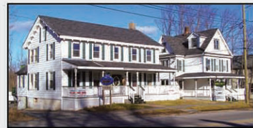
Monticello Investment Property $779,900 Attractive 8-unit (comm/res) in fabulous location! Everything updated within the past 3-years. Paved parking in rear. Professional offices surround. Near Gov't Center, retail, gas, banks, schools, etc... Just moments from the Racino. #18866
